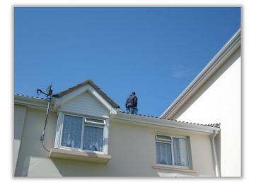
Two men were working on this roof cleaning moss from the surface of the roof tiles. No edge protection had been provided, with the only safety measure adopted being a rope tied around one of the men's waist held by the other man sitting on the ridge of the roof.
