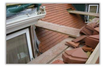
A Prohibition Notice was served preventing further use of this access platform following an accident where an operative had fallen whilst working on the roof.
